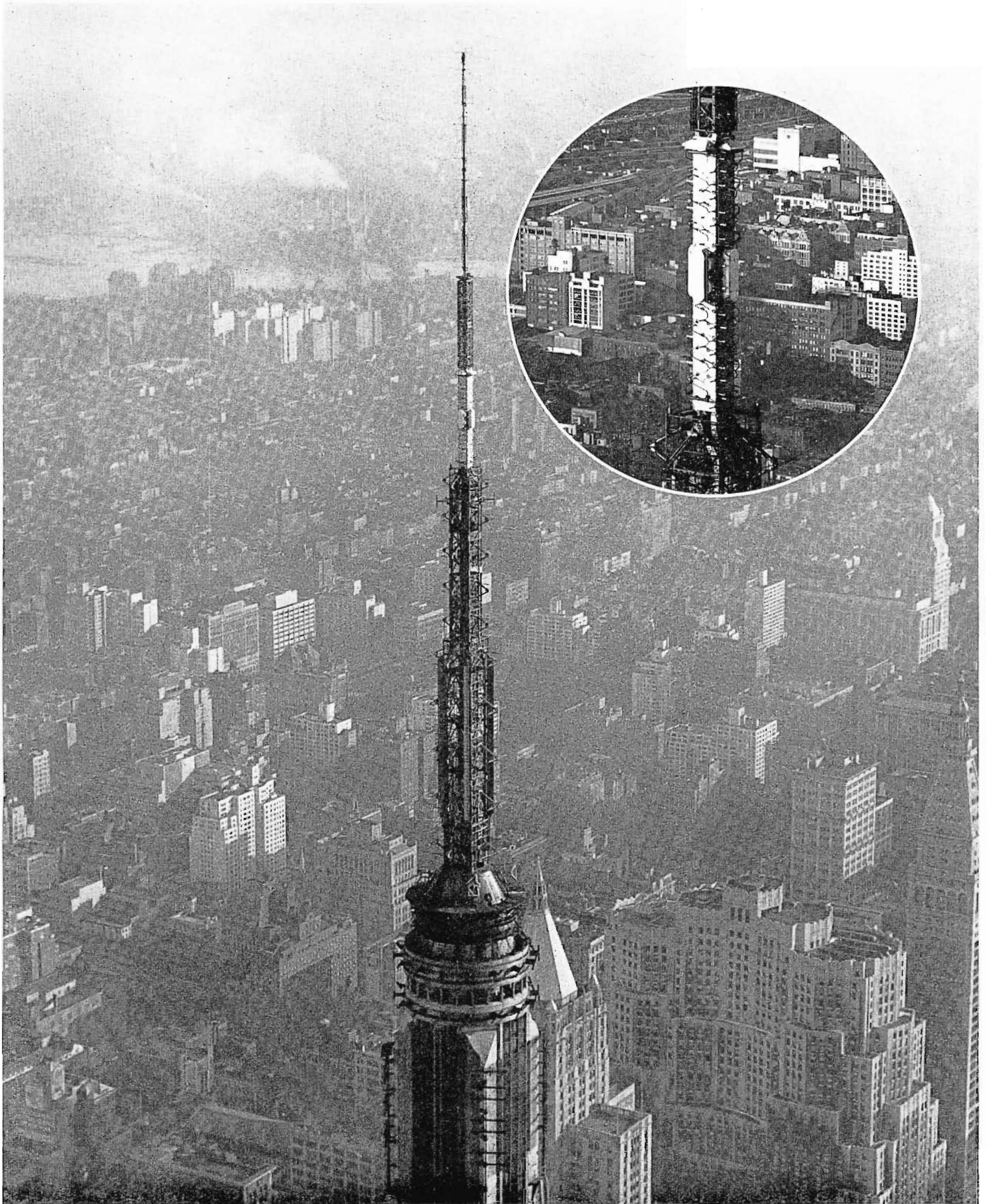
FIG. 1. Helicopter view shows "new look" of multiple antenna structure on Empire State Building, which now includes WABC-TV's gleaming new RCA Zee Panel.
